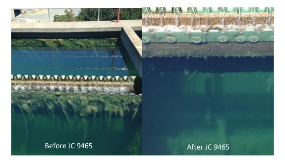
As you can see, we were able to remove significant quantities of algae and biofilm deposits. This potable water treatment plant saw other significant improvements: improved filtered water turbidity, lower chlorine consumption, lower THM's formation, longer filter run time between backwashing, and lower treatment cost. If you are interested in our new chemical solution, please check out our website or contact us for more information.
