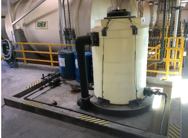
Figure 4 – Chemical Storage Area and Containment Area for JC9450
