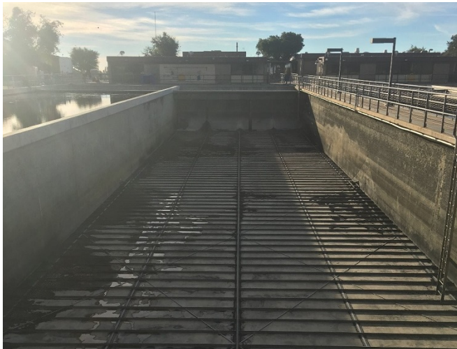
Figure 6 – A drained and cleaned treatment basin
